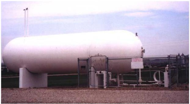
Top, A 18,000-gallon propane tank similar to the one that exploded at the Herrig Brothers Feather Creek Farm (the turkey farm) in Albert City, Iowa, from NIOSH report. Note protective fencing around piping for this tank which was lacking at the Iowa farm propane tank.
